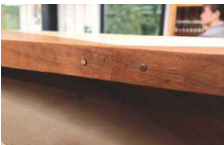
▲ Pic.45 As a closing mechanism, I used simple little magnetic pins, which produce a nice 'click' when closing the doors
